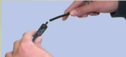
a. Fit drippers to dripper line
